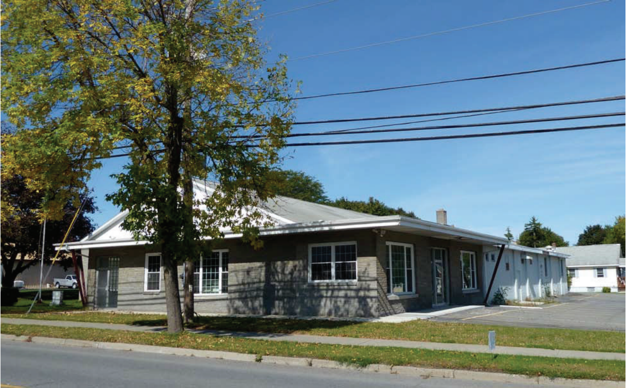
The former Knights of Columbus Hall viewed from the south side of Main Street in Ravenna. It has load-bearing masonry walls and wood truss main roof structure.
