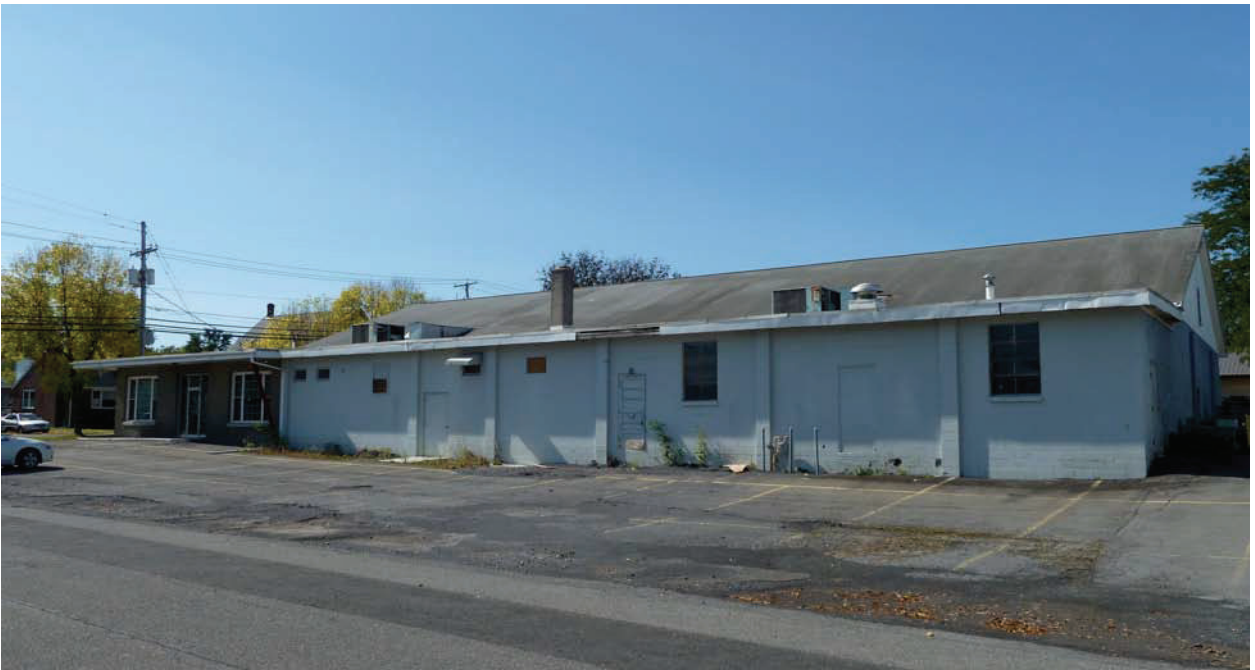
View from the east showing site area available for parking.
